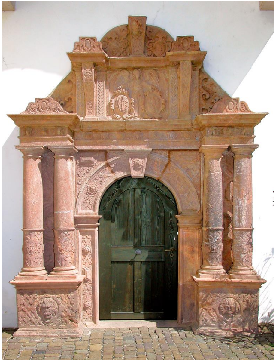
IMAGE 14: This decorative entrance is carved from pink, rhyolitic Tuff. It is the front of a church at Colditz Castle, Germany.
